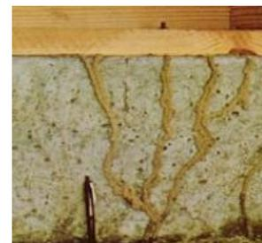
picture on the left), as well as conditions conducive to termite and other WDO infestation (such as wood that is too close to the ground, dead tree stumps by the house, improper grading, leaky gutters or downspouts, or tree branches overhanging or touching the home). The inspector will also look for evidence of infestation by other wood-destroying insects.
